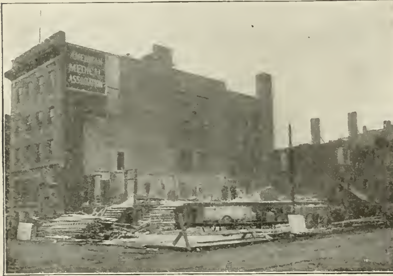
Fig 4—Wrecking the old buildings.
