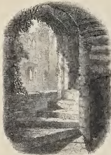
STAIRCASE IN GWENT TOWER.
