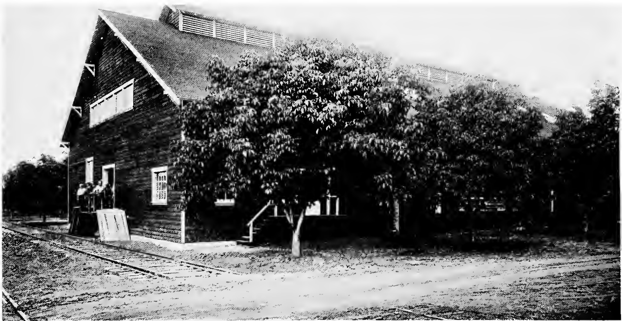
(ABOVE) THE ASSOCIATION'S PLANT AT SANTA ANA IS AS EFFICIENT AS IT IS PLEASING TO THE EYE (BELOW) THE IRVINE PLANT IS MODERN IN EVERY RESPECT
