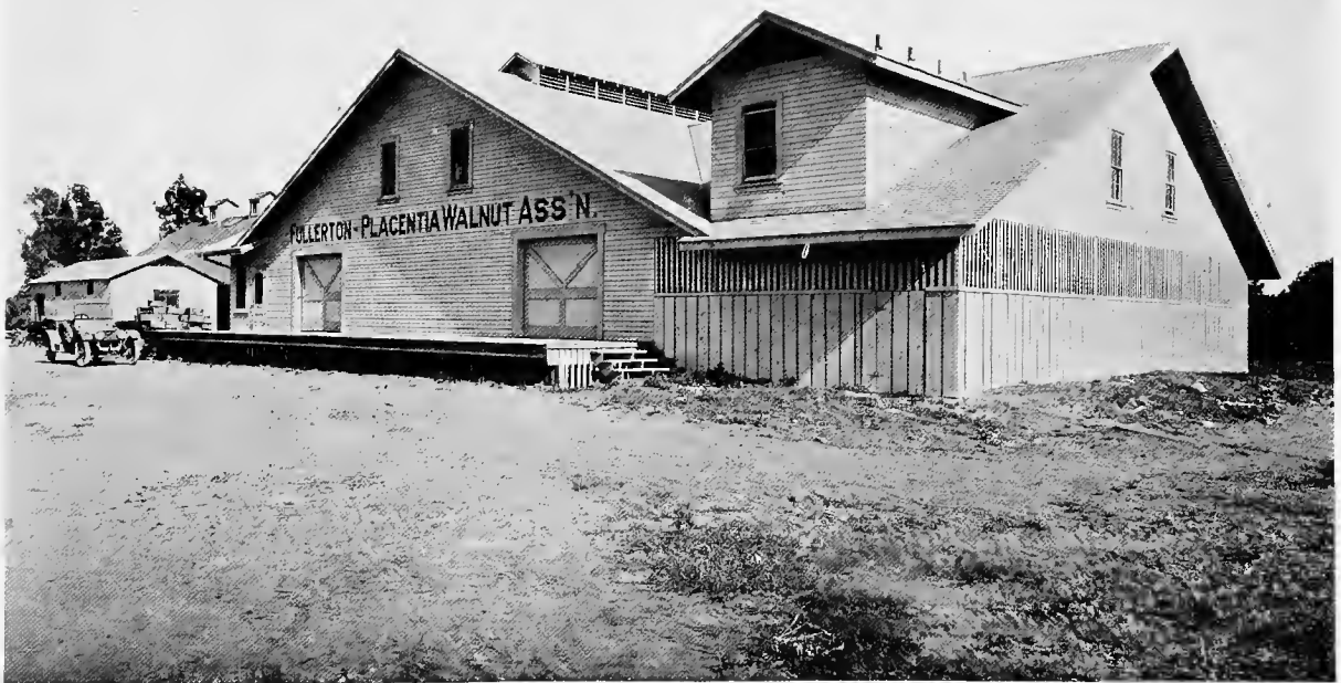
(ABOVE) THE SANTA BARBARA PLANT IS ONE OF THE MOST MODERN AND EFFICIENT (BELOW) FULLERTON GROWERS MAKE THEIR HEADQUARTERS HERE
