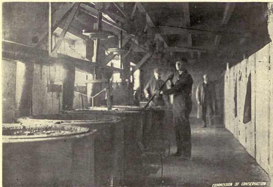
Rendering Room where the Fish Waste was Treated to Separate the Valuable Oil Content, Port Dover, Ont.
