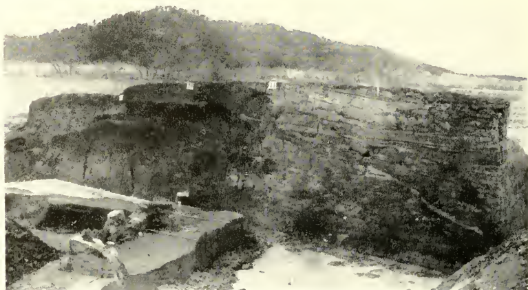
A , Profile L-1, showing the various stages of construction.
