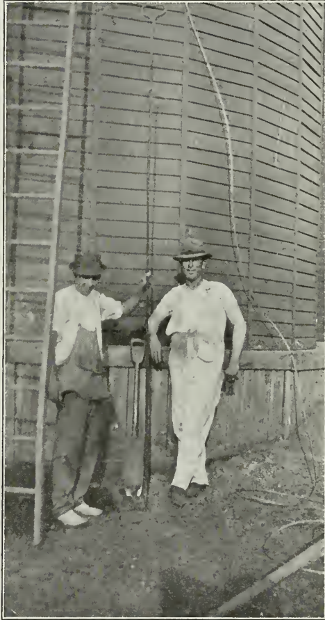
FIG. 37.—The drill (in left hand) used in making groundings.
