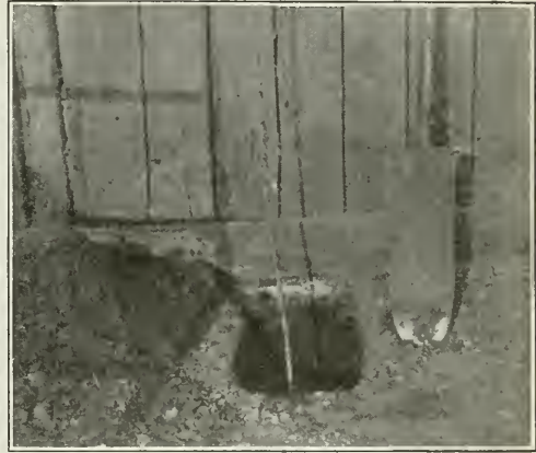
FIG. 39.—Ground rod down 10 feet.
