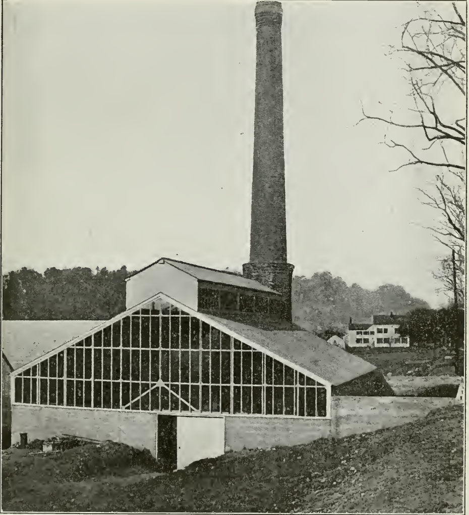
Boiler Room Located so as to Minimize Hauling Operations.
