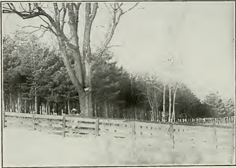
Fig. 10 illustrates a plantation of Scotch Pine made about twenty-five years ago. This was a gravelly hillside of small value for cultivation. At a very small cost it was replanted, and to-day is a valuable asset to the farm.
