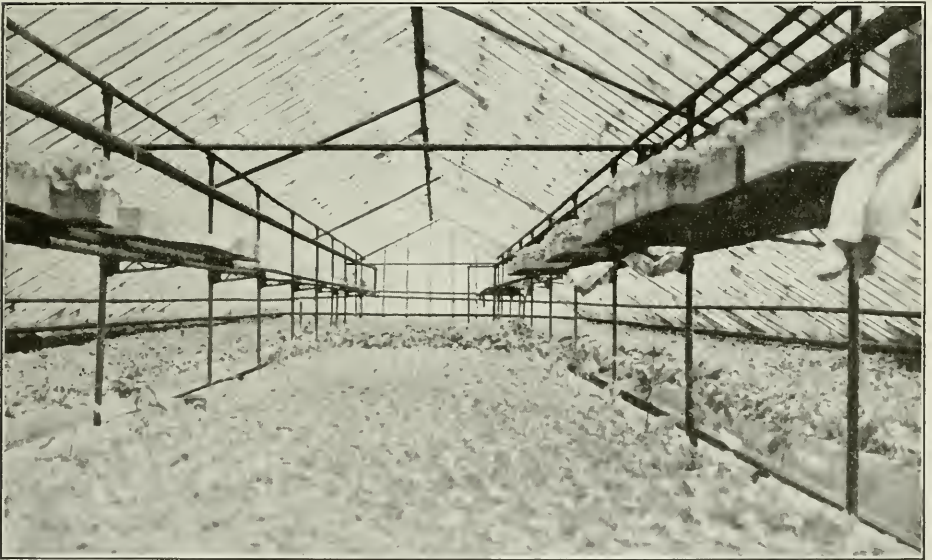
Raised benches are necessary where rhubarb is forced. In narrow pipe frame houses iron supports are often clamped to the supports to make a shelf for early plant boxes.
