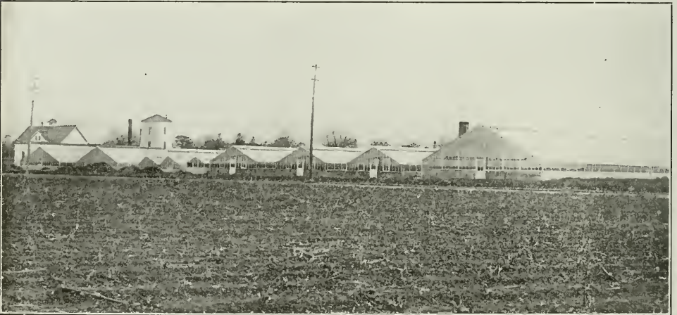
Previously only narrow, low roofed houses were used, but wider ones are now the only ones in demand. The change from 14 ft. to 75 ft. houses can plainly be seen here.
