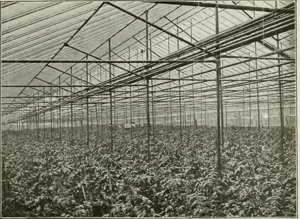
Pipe frame construction, showing the network of pipes necessary to insure safety. Compare these views with the one on the next page.
