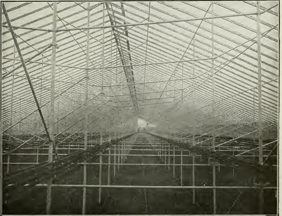
Interior of largest pipe frame greenhouse in Canada
