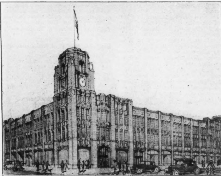
Like many outstanding newspaper business of recent years, the new Chronicle building is an excellent example of "industrial Gothic" architecture.
