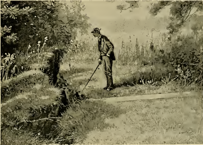
AN EFFECT OF THE EARTHQUAKE AT CHARLESTOWN
