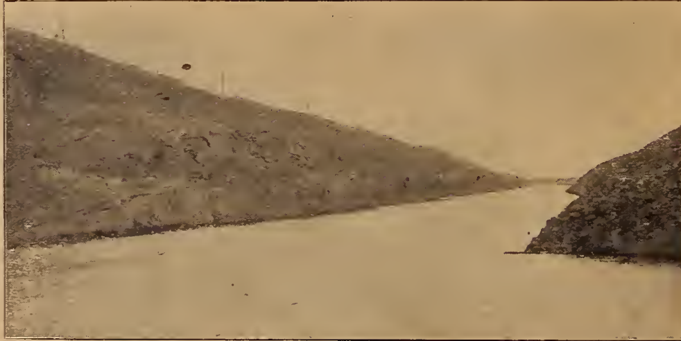
DEEP CUT IN MAIN CANAL
