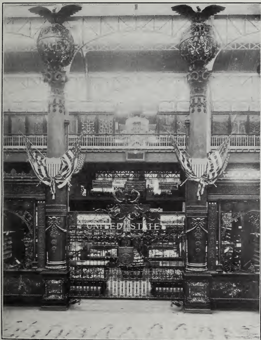
H-2. MAIN ENTRANCE, SHOWING CLOSED PORTCULLIS, DEPARTMENT OF MINING AND METALLURGY.
