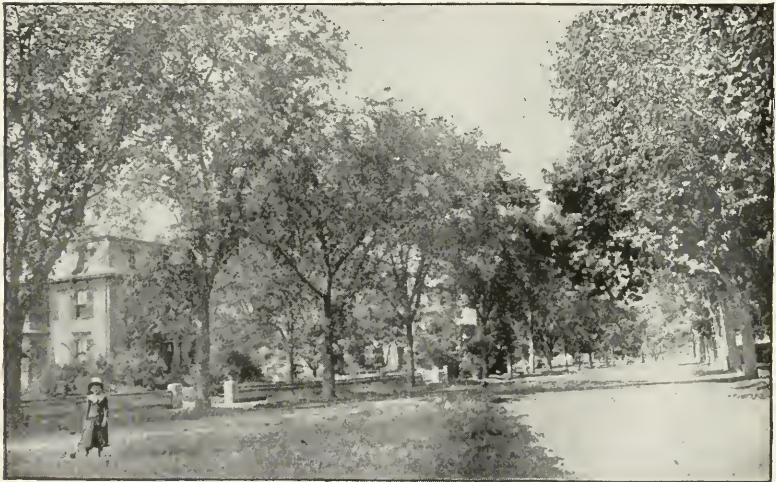
MONUMENT ST., LOOKING NORTH.
