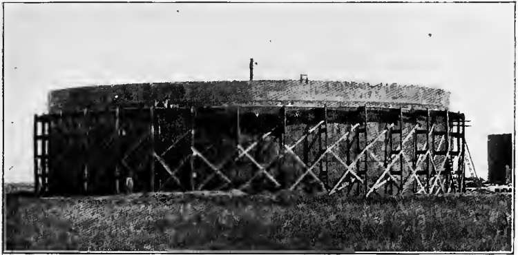
PLATE 21.—A fifty-thousand barrel storage tank for petroleum in course of construction.
