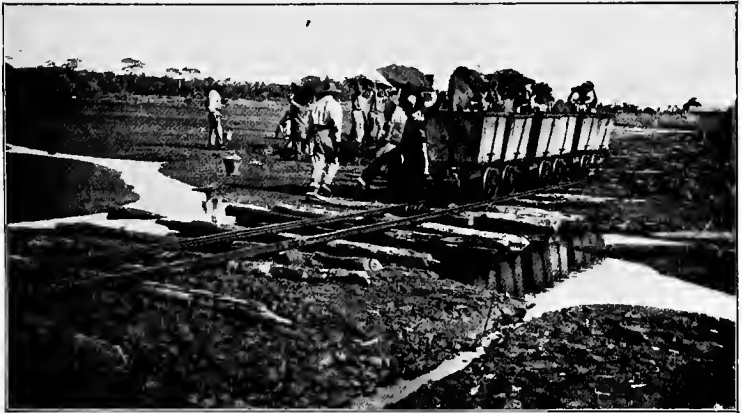
PLATE 18.—Great Pitch Lake at Trinidad. Showing the pitch being excavated and loaded into trucks.
