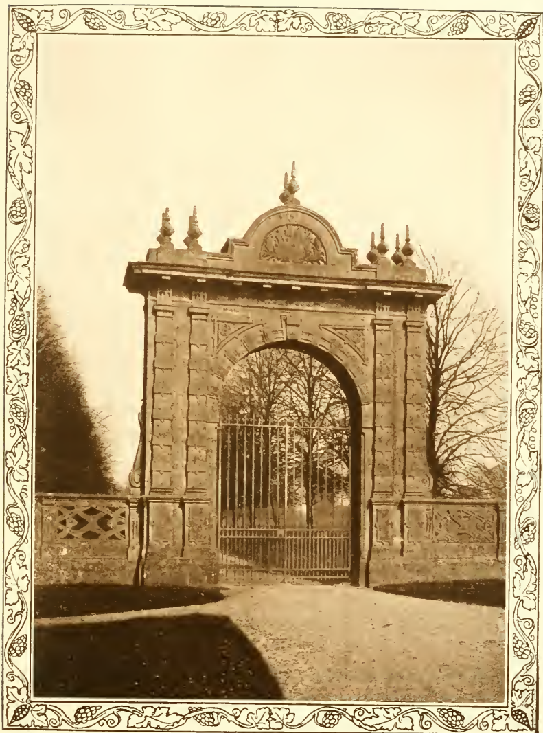
ENTRANCE TO CHARLECOTE PARK
