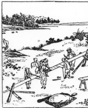
FIG. 13.—PREPARING LINING TUBES.
