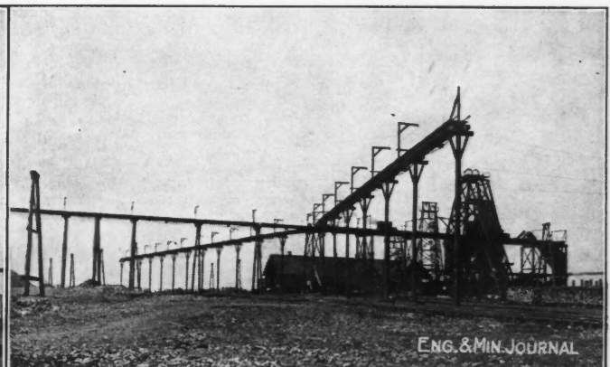
STOCKPILE CLEANED UP Trestle leading to left is of old two-leg type.
