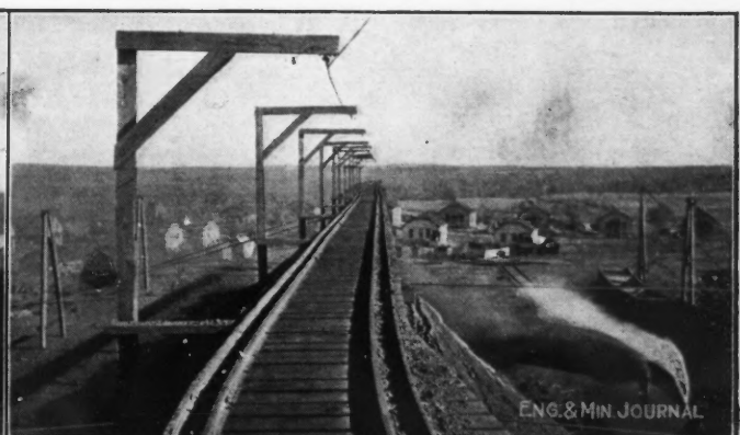
TOP OF TRESTLE
