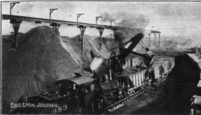
SHOVEL AT WORK ON FIRST CUT
