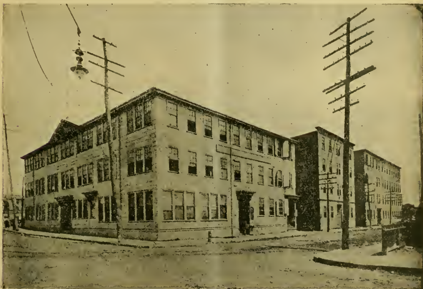
FIG. 1. — THE THREE RUINED FACTORIES, BEFORE THE EXPLOSION. (The Harney building is on the right.)
