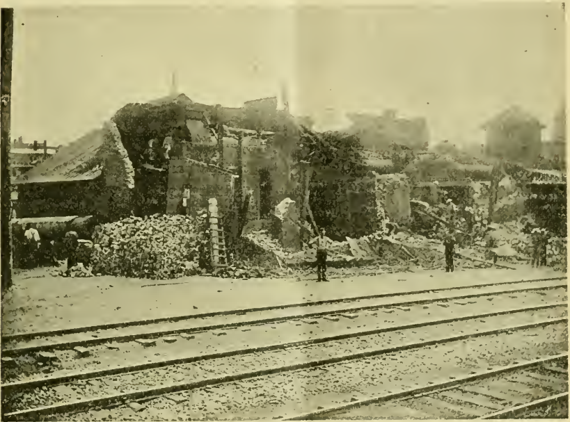
FIG. 3.—GENERAL VIEW OF THE DESTROYED POWER PLANT.
