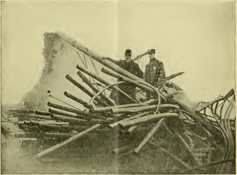
FIG. 5. — SHOWING THE TUBES OF THE EXPLODED BOILER.
