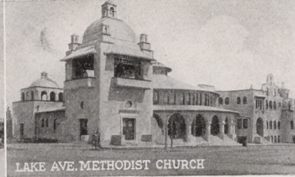
LAKE AVE. METHODIST CHURCH
