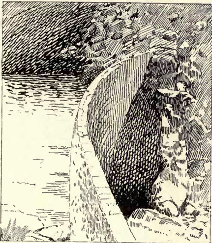
Bear Valley Arched Masonry Dam, California.
