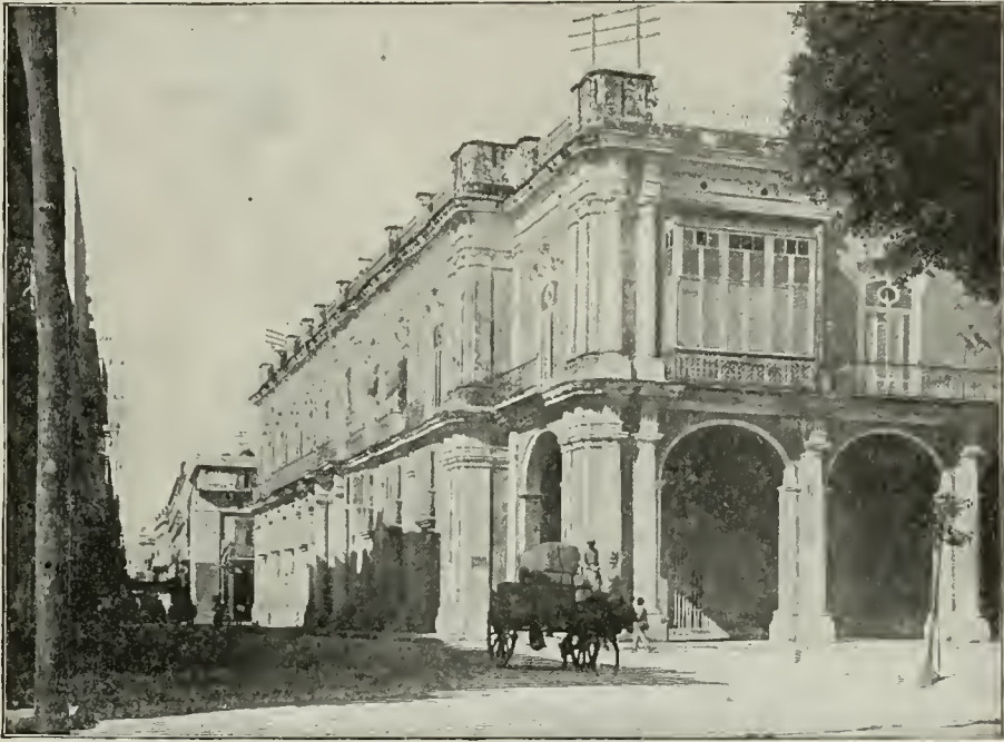
GOVERNOR-GENERAL'S PALACE, HAVANA.—OFFICIAL RESIDENCE OF CAPTAIN-GENERALS WEYLER AND BLANCO.—From a Photograph.
