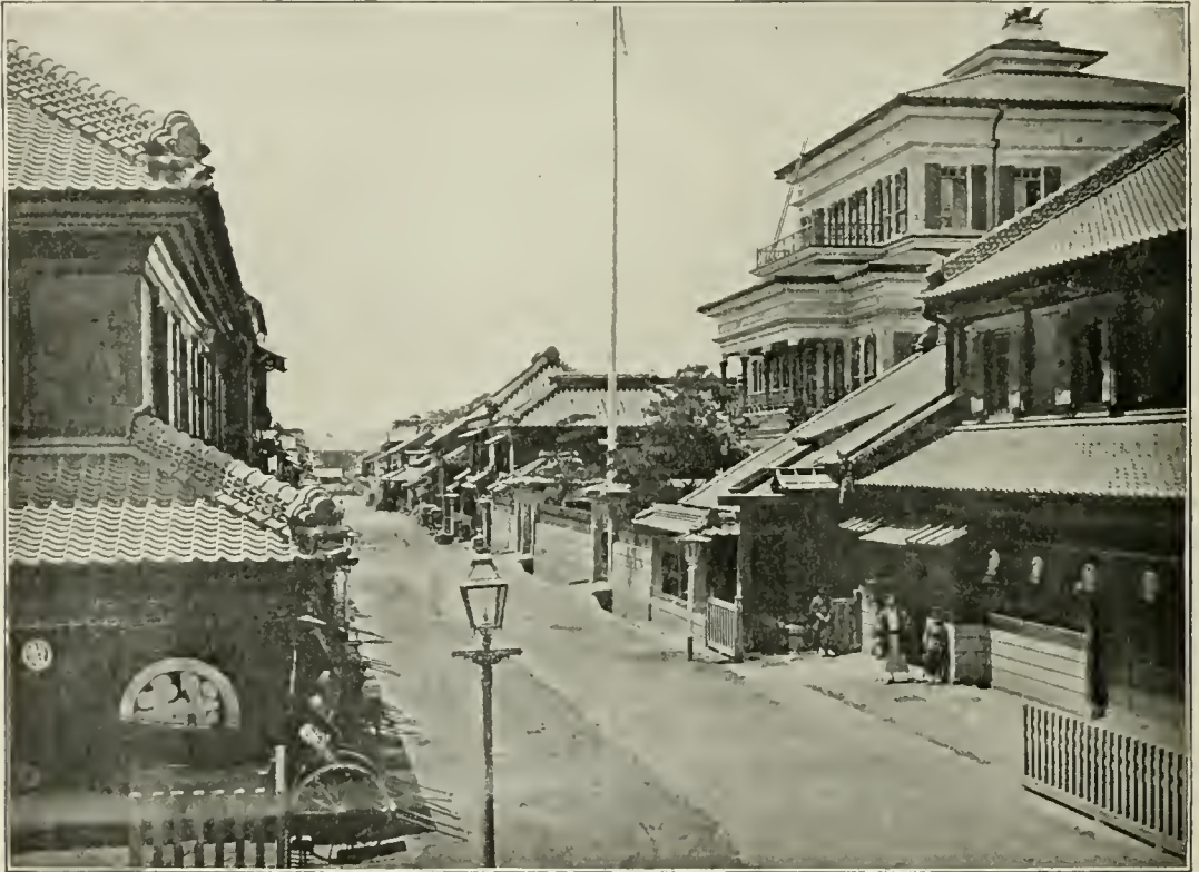
STREET SCENE IN TOKIO—MITSUI BANK.—From a Photograph.
