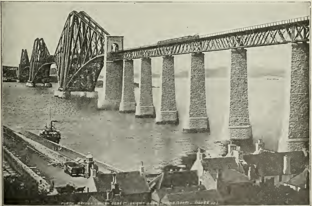
CANTILEVER BRIDGE OVER THE FRITH OF FORTH.
