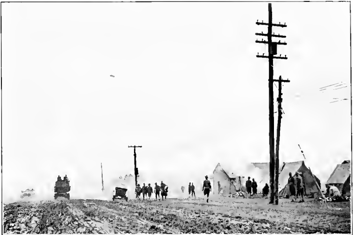
TELEPHONE CONSTRUCTION AT CAMP MILLS, GARDEN CITY, LONG ISLAND
