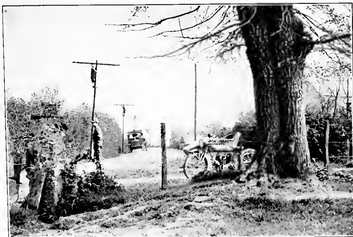
STRINGING WIRE FROM ST. NAZAIRE TO NANTES
