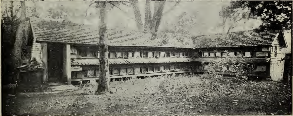
FIG. 1.—WEST SIDE OF THE BEE-HOUSE.
