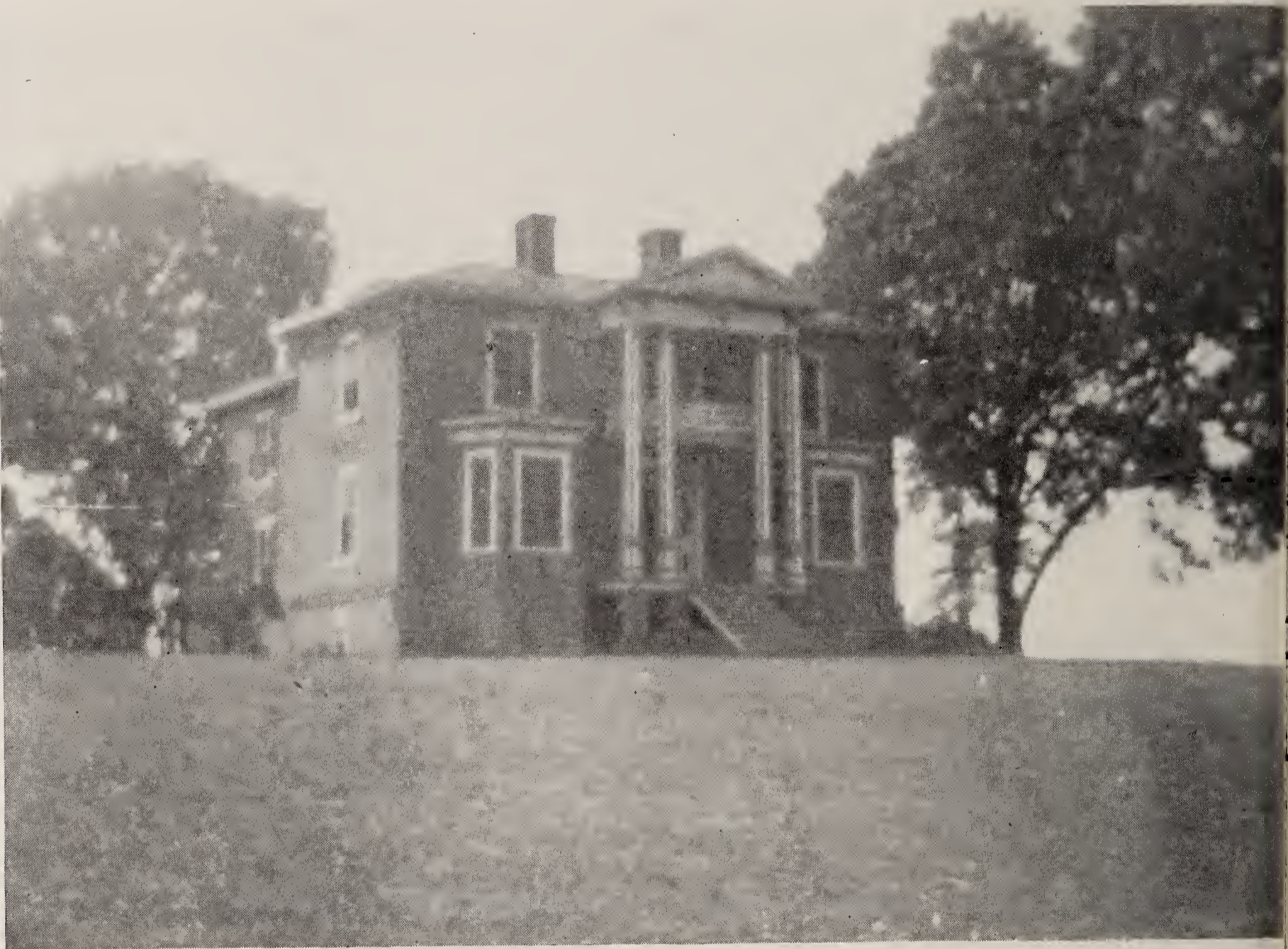
"HUNTSMAN'S REST", ORANGE COUNTY, VA. Home of Joseph Miles Henderson and Hannah Irving Terrill. Destroyed by fire in 1930.
