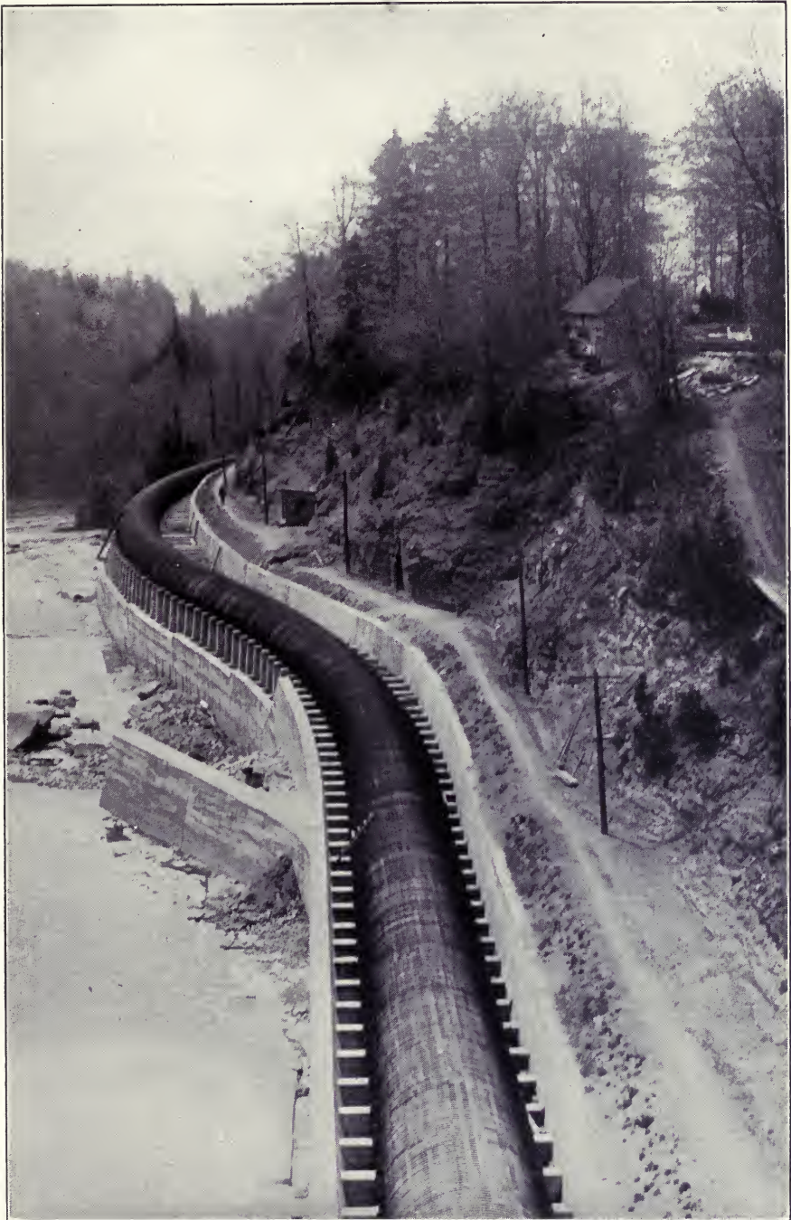
WOOD STAVE PIPE LINE, TRENTON FALLS STATION
