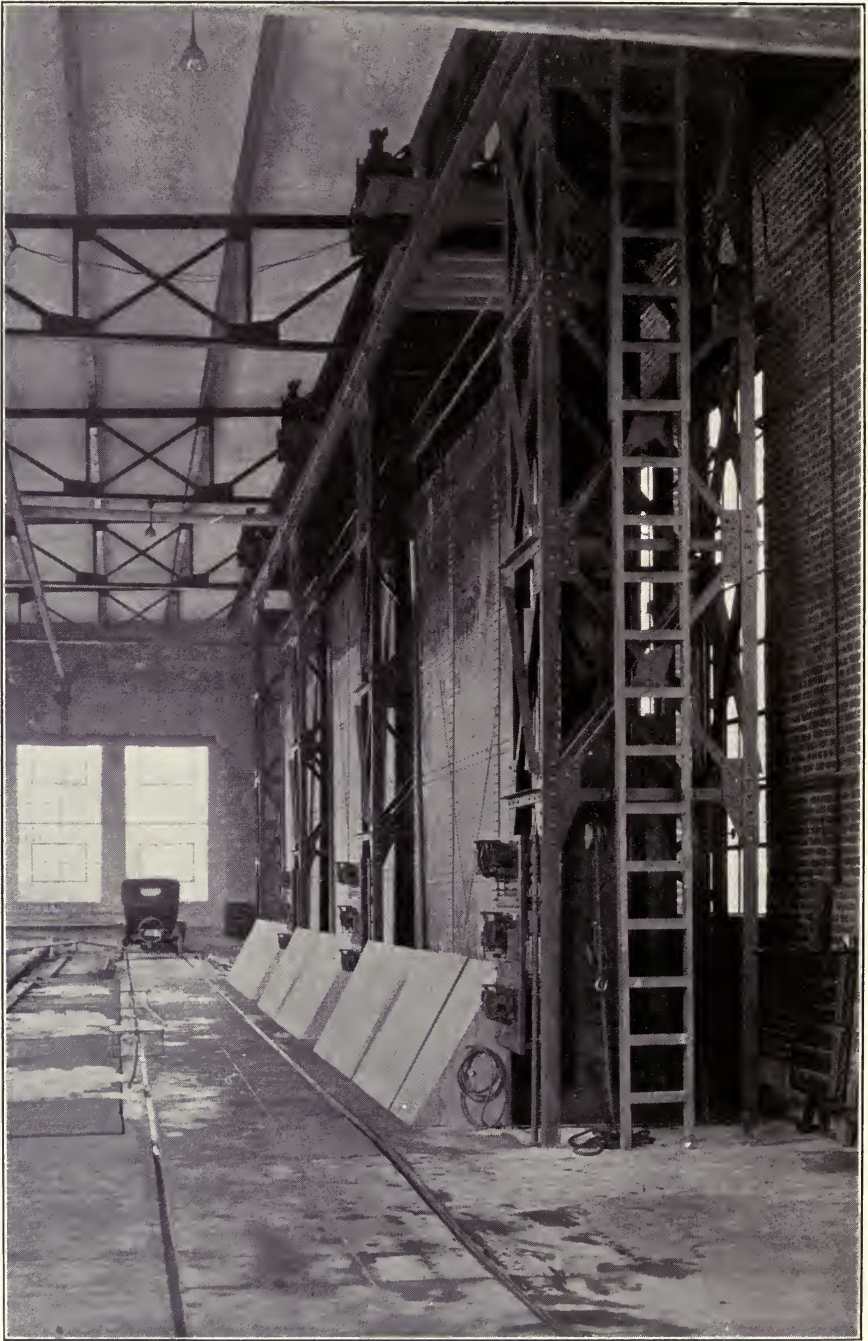
INTERIOR OF GATE HOUSE, COHOES STATION
