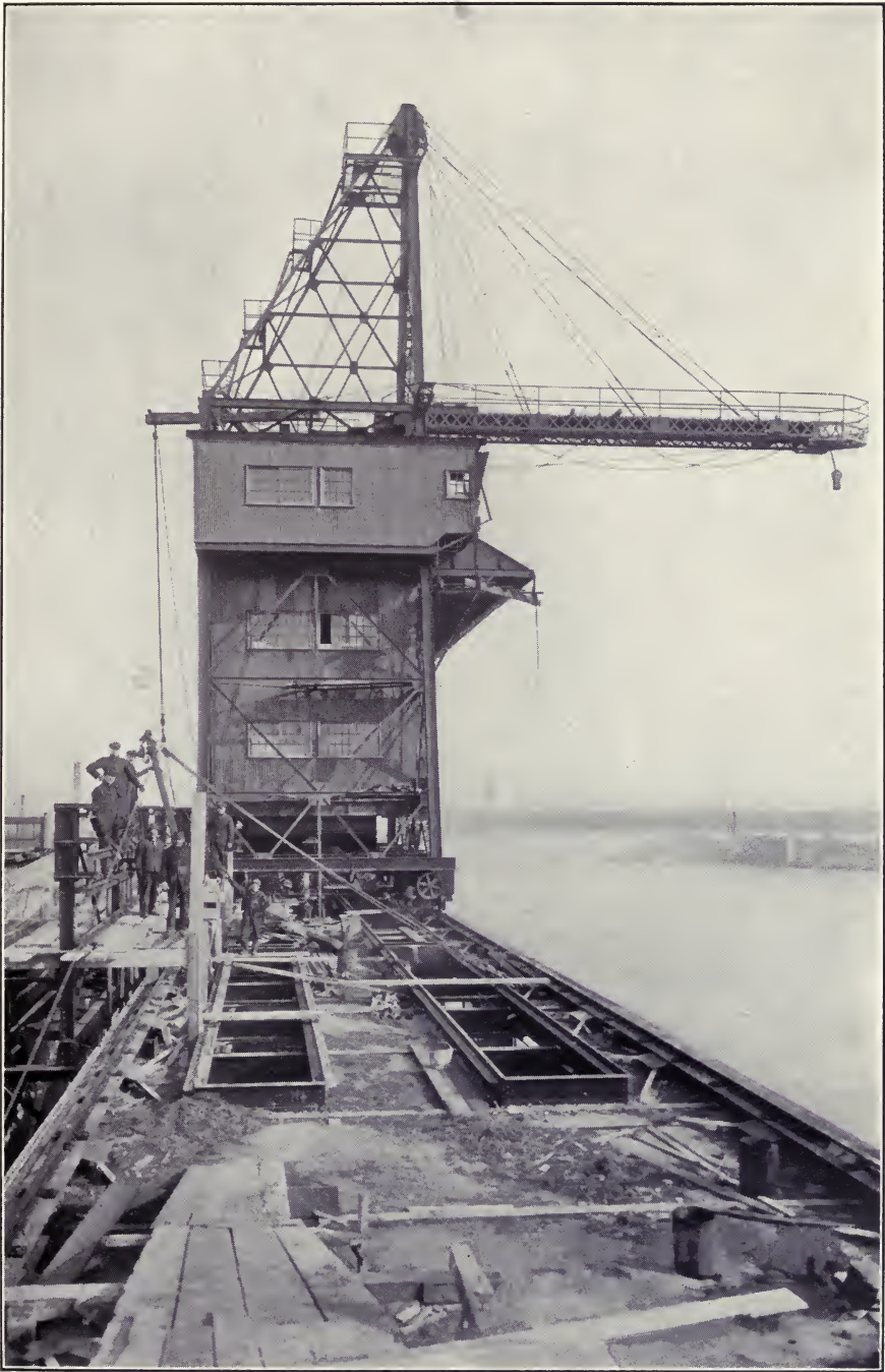
TRAVELING COAL TOWER, HELL GATE STATION
