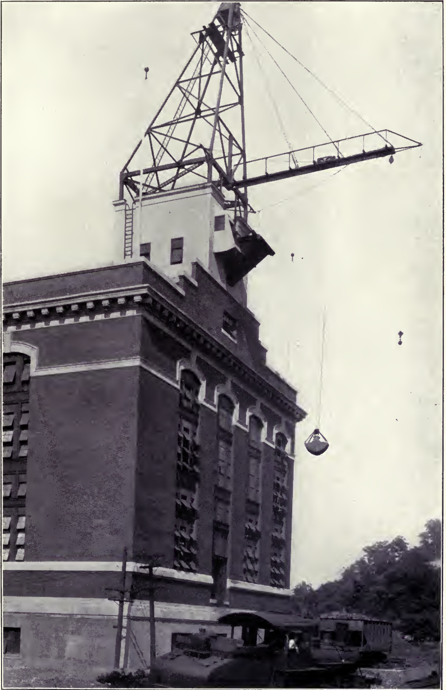
COAL HANDLING TOWER, MILLERS FORD STATION
