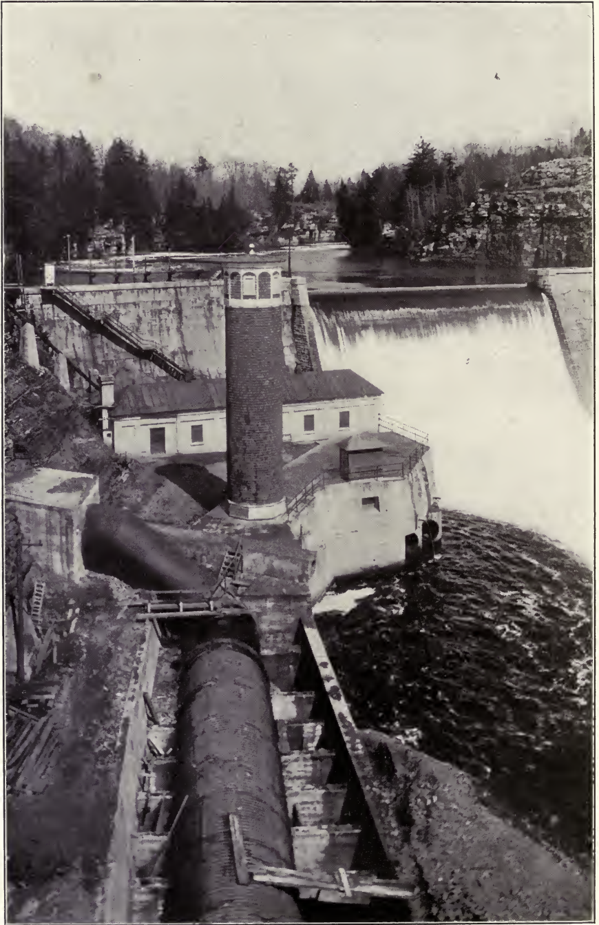
DAM, TRENTON FALLS STATION.
