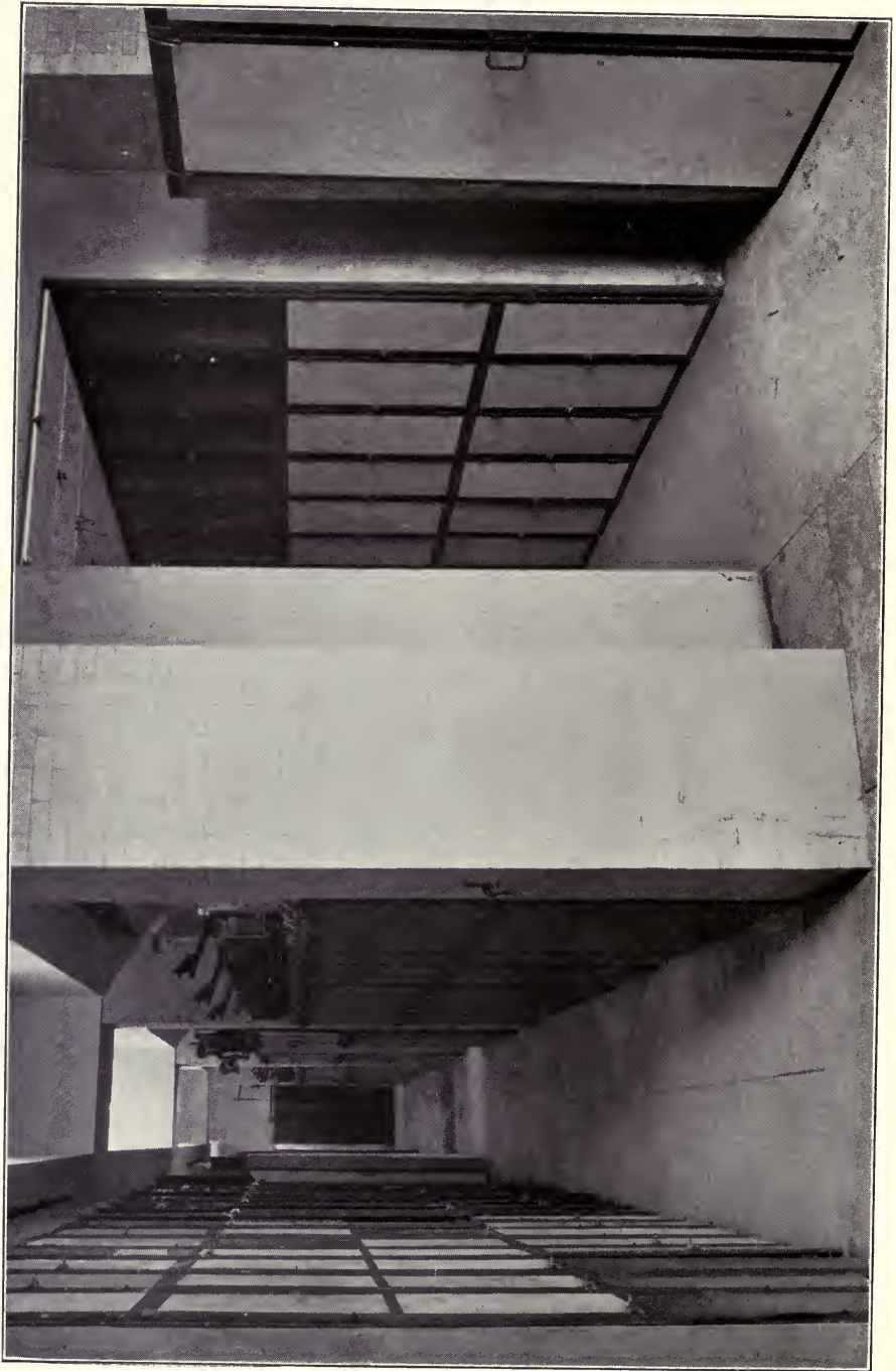
SWITCH COMPARTMENTS, SHERMAN CREEK STATION
