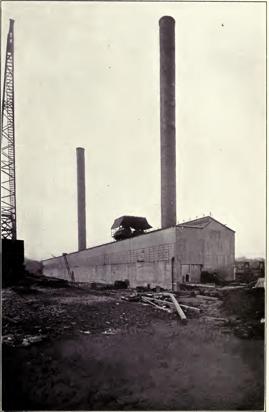
BOILER HOUSE, UNITED STATES GOVERNMENT EXPLOSIVES PLANT "C"
