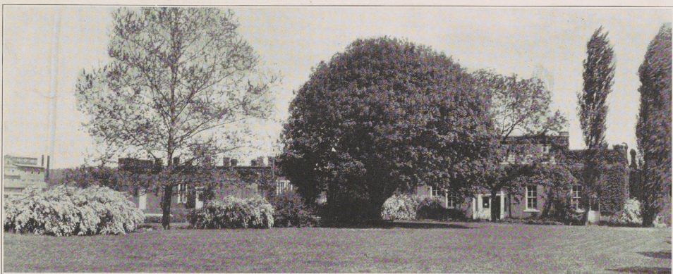
NEOSHO NURSERIES—View of Office and Packing Houses From the South, Neosho, Missouri
