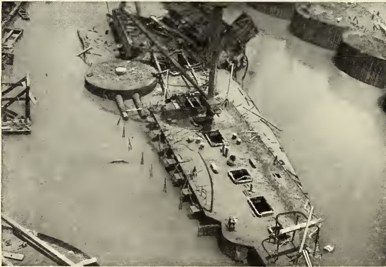
THE AFTER-DECK OF THE "MAINE," UNCOVERED AS THE WATER WAS PUMPED OUT OF THE COFFER-DAM.
