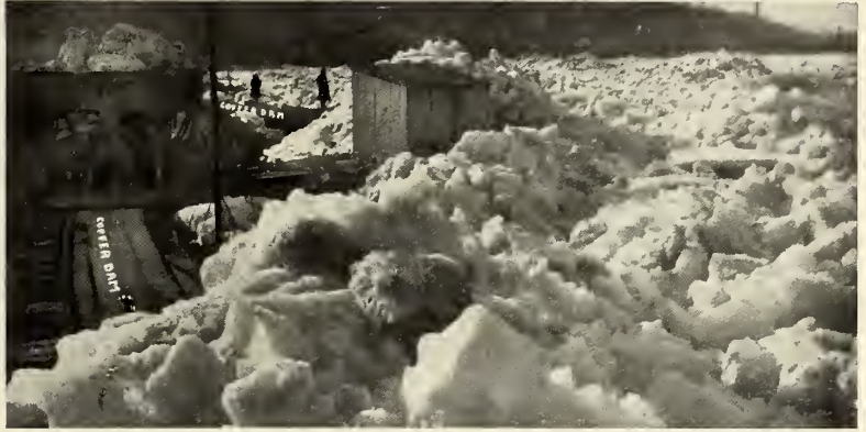
A MOUNTAIN OF ICE THREATENING TO OVERWHELM THE COFFER-DAM.
