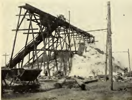
A PILE OF SALT UNDER THE WASHER AND STACKER, READY FOR SHIPMENT.
