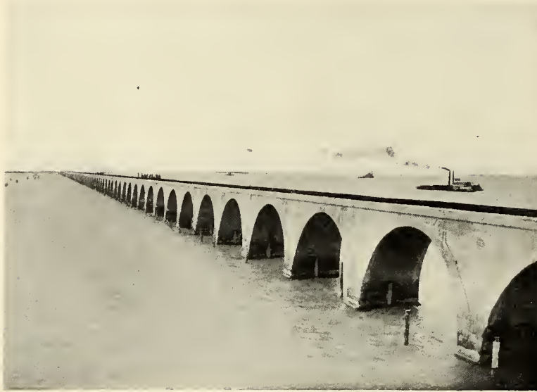
A CONCRETE CENTIPEDE REACHING ACROSS THE SEA.
