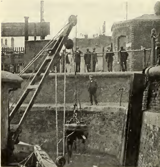
AN ELECTRO-MAGNET LIFTING SCRAP-IRON FROM THE BOTTOM OF THE RIVER THAMES.
