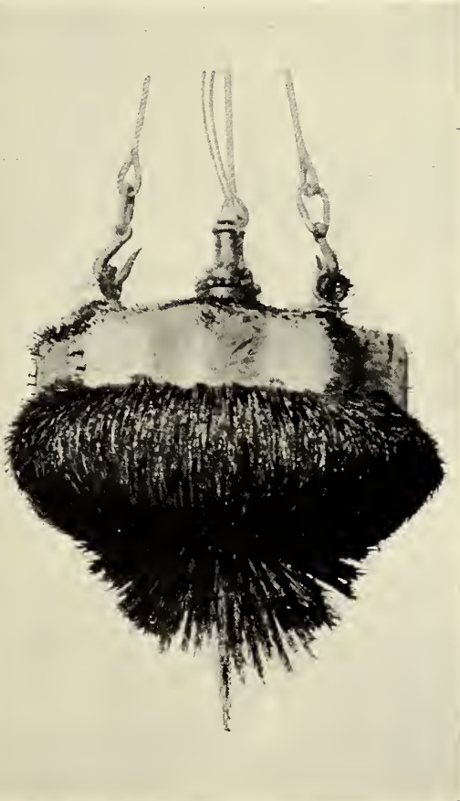
AN ELECTRO-MAGNET LOADED WITH SWEEPINGS FROM A MACHINE-SHOP.
