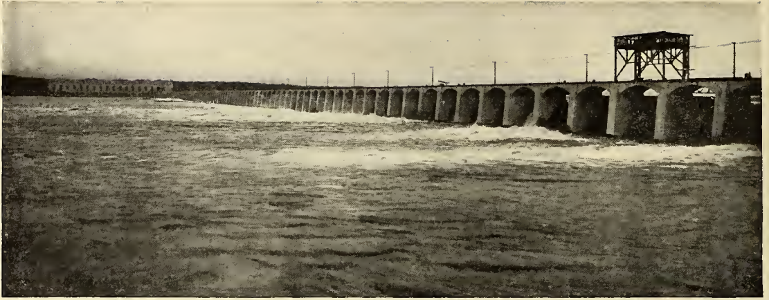
THE COMPLETED KEOKUK DAM, SHOWING THE TRAVELING CRANE WITH WHICH THE GATES ARE OPENED.
