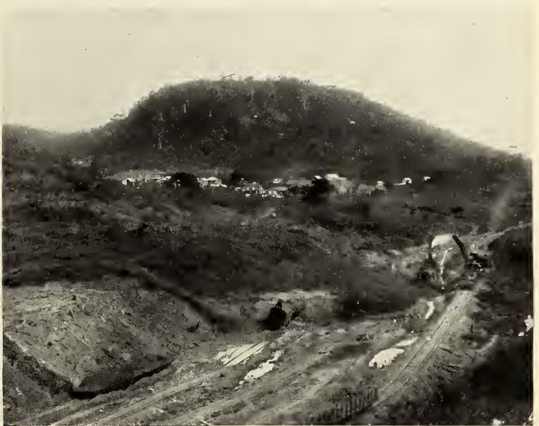
THE CUCARACHA SLIDE MAKING MORE WORK FOR THE CANAL DIGGERS.
