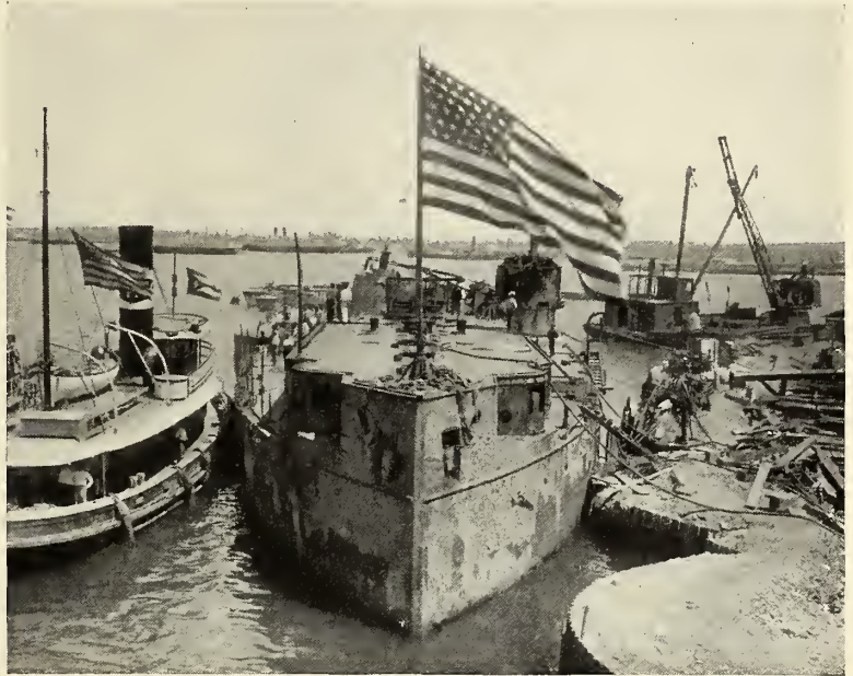
THE AFTER PORTION OF THE "MAINE" FLOATED OUT OF THE COFFER-DAM AND READY TO BE BURIED AT SEA WITH HONORS.
