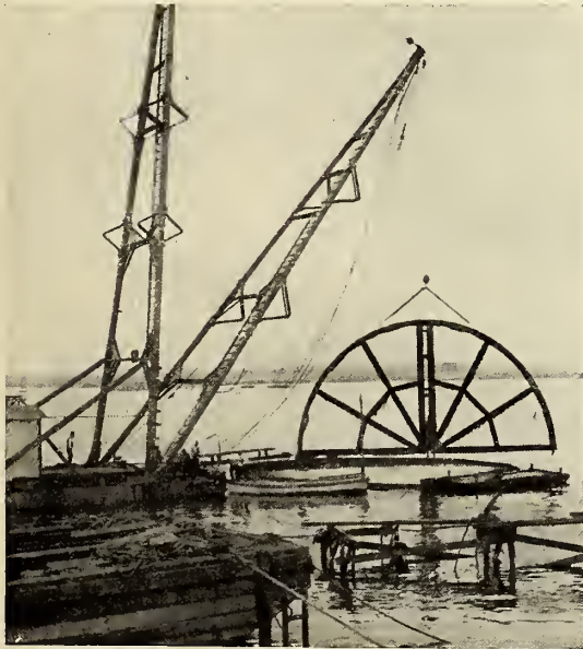
LIFTING HALF A TEMPLET OUT OF A COMPLETED CYLINDER.
