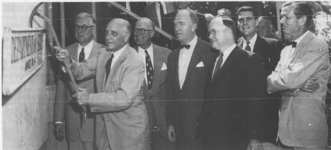
Deputy under secretary Loy W. Henderson begins demolition of temporary building
