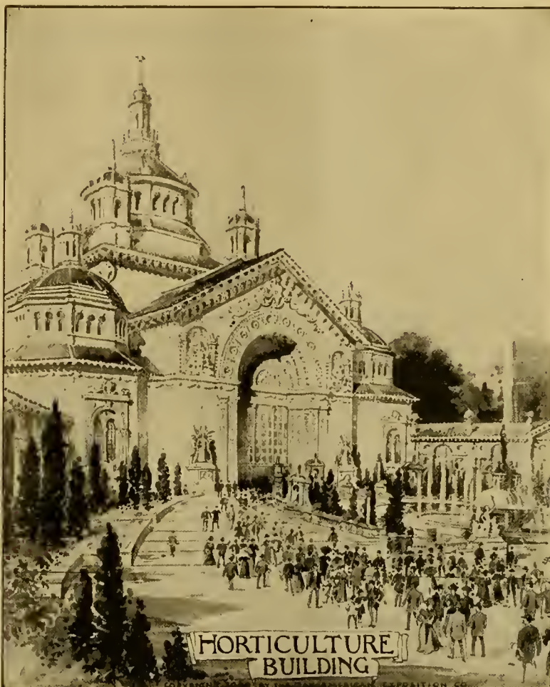
ENTRANCE TO HORTICULTURAL BUILDING, PAN-AMERICAN EXPOSITION.
