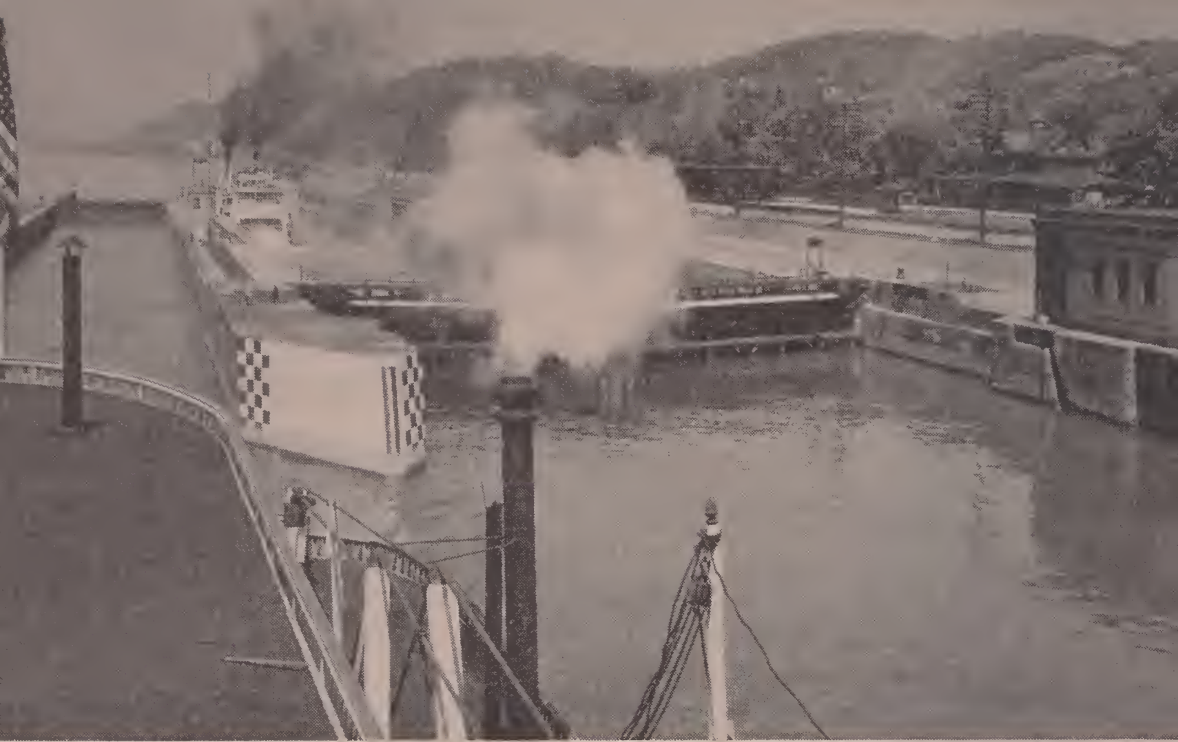
LOCK AND DAM
