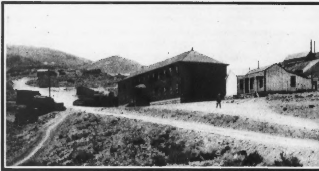
BOARDING HOUSE AT THE EUREKA CONSOLIDATED
