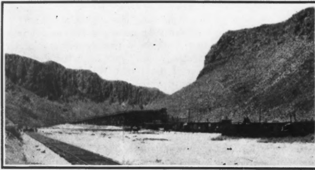
ORE TRANSFER STATION AT PALISADE
