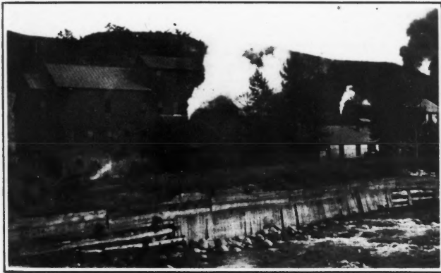
FIG. 3. WASHERY AT NORTHERN PACIFIC MINES
