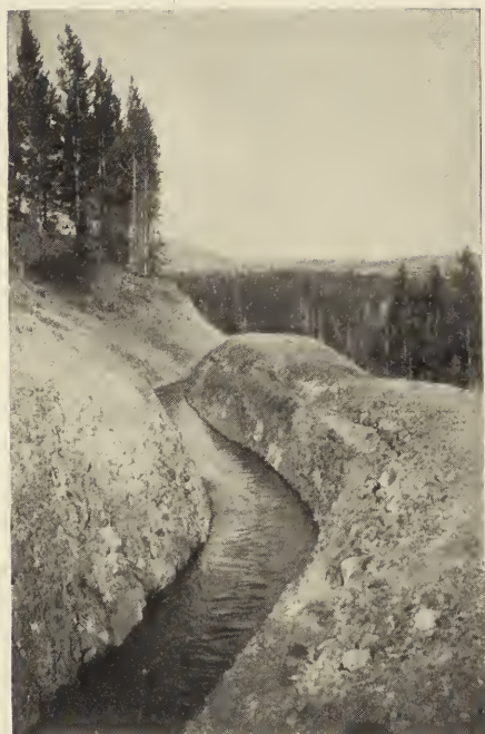
COMPLETED DITCH AT HORSE-SHOE BEND.
