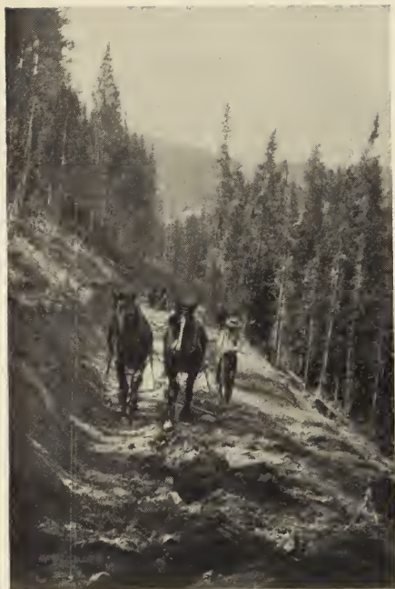
PLOWING ON GRADE LINE.
