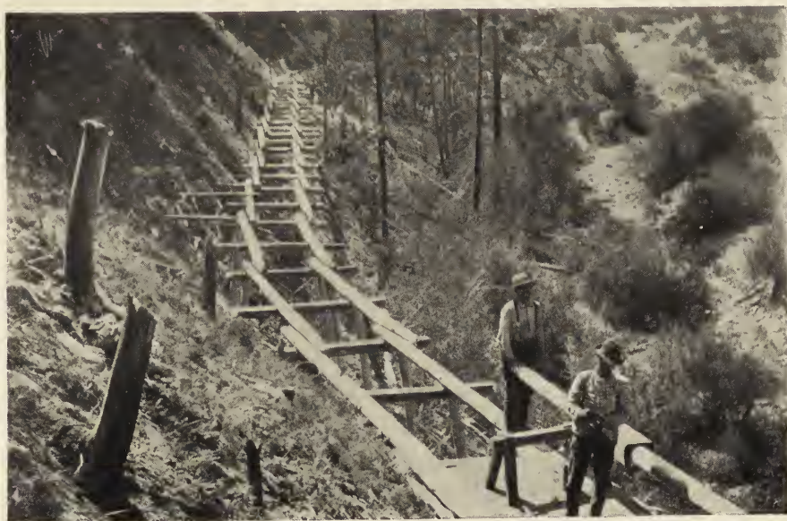
TRESTLE CONSTRUCTION, RAPP'S CREEK DITCH, IDAHO.
