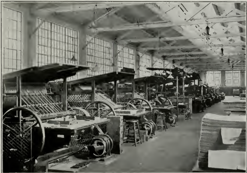
NORTH WING OF THE NEW PRESS-ROOM
