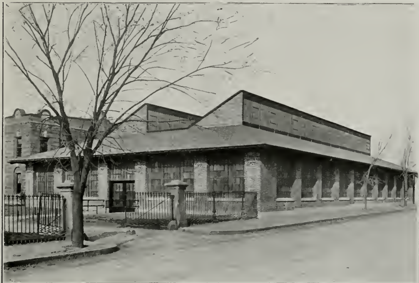
THE NEW PRESS-ROOM BUILDING
