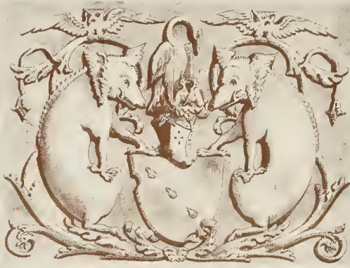
BRICK PANEL. WEST FRONT.
