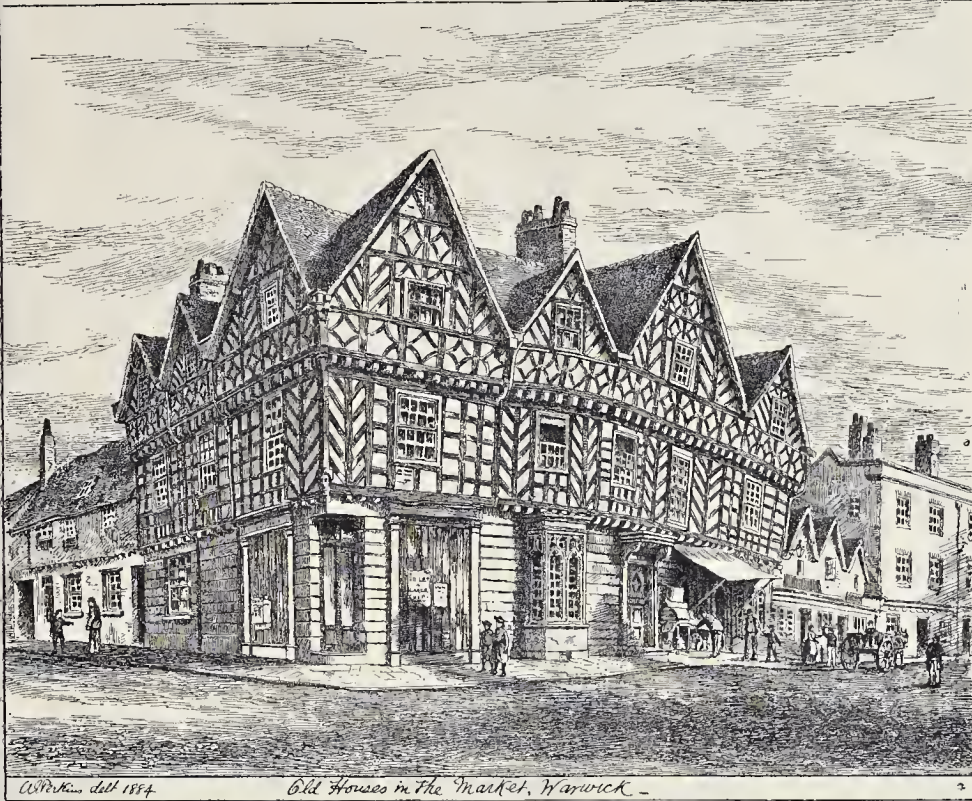
Old Houses in The Market, Warwick -
