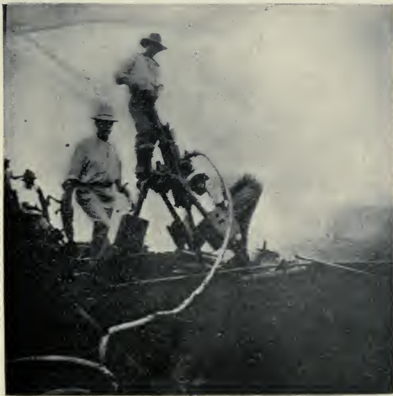
DRILLING AT CULEBRA CUT (1908)
