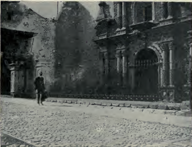
STREET AND CHURCH FAÇADE, AREQUIPA
