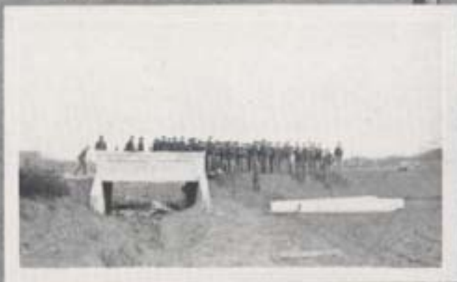
Class in road and bridge construction
