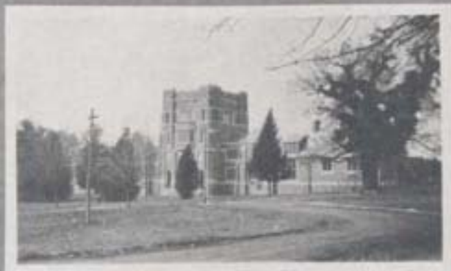
The McBryde Bldg. of Mechanics Arts
