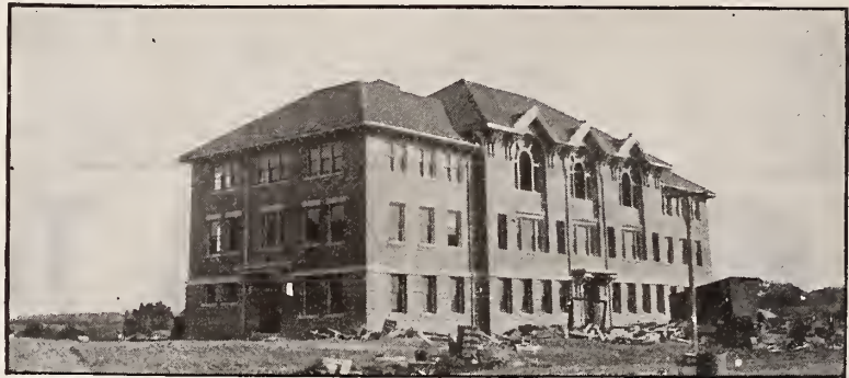
ANOTHER VIEW OF NEW YORK STATE POULTRY HUSBANDRY BUILDING. Cost complete will be $90,000. Is a part of New York State College of Agriculture. Dimensions are, 132 feet in length, 48 feet in width in the central portion and 37 feet in width at the ends. Height, three full stories.
