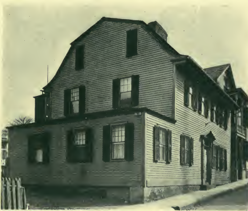
HOUSE AT NUMBER 36 CHURCH STREET, NEWPORT, RHODE ISLAND.
