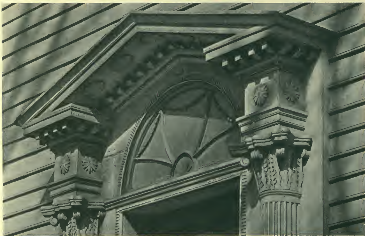
DETAIL OF DOORWAY—NUMBER 228 SPRING STREET, NEWPORT, RHODE ISLAND.
