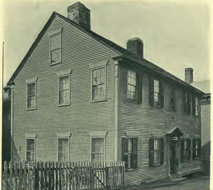
HOUSE AT NUMBER 27 CHURCH STREET, NEWPORT, RHODE ISLAND.
