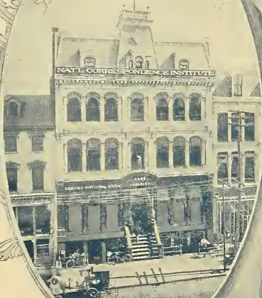
View from Post office Department.
