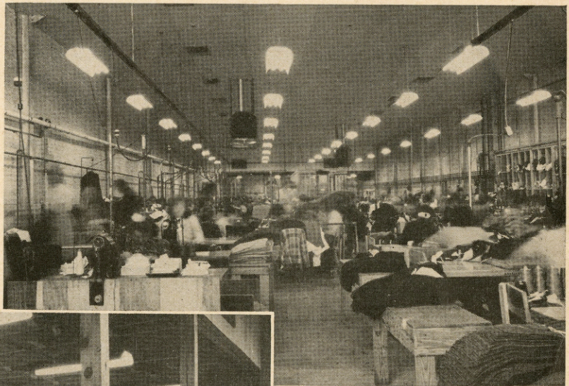
A PLANNED lighting system overcame the illumination defects simply, economically, and attractively, as these two pictures show. In the pants department, seen above, four rows of modern fluorescent lights supply some 25 foot-candles of even, eye-easy illumination. (The blurs in the picture were caused by quick movements of the women workers as they pursued their specialized operations.) The coat, vest and pressing departments have been similarly re-lighted for more efficient production. The special-order department is pictured at left. Sight-soothing illumination speeds the manufacture of uniforms for police, guards and other purposes, in this busy section.
