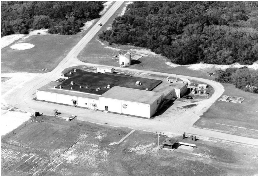
Figure A-18. Aerial view of the MCC, February 21, 1996.
