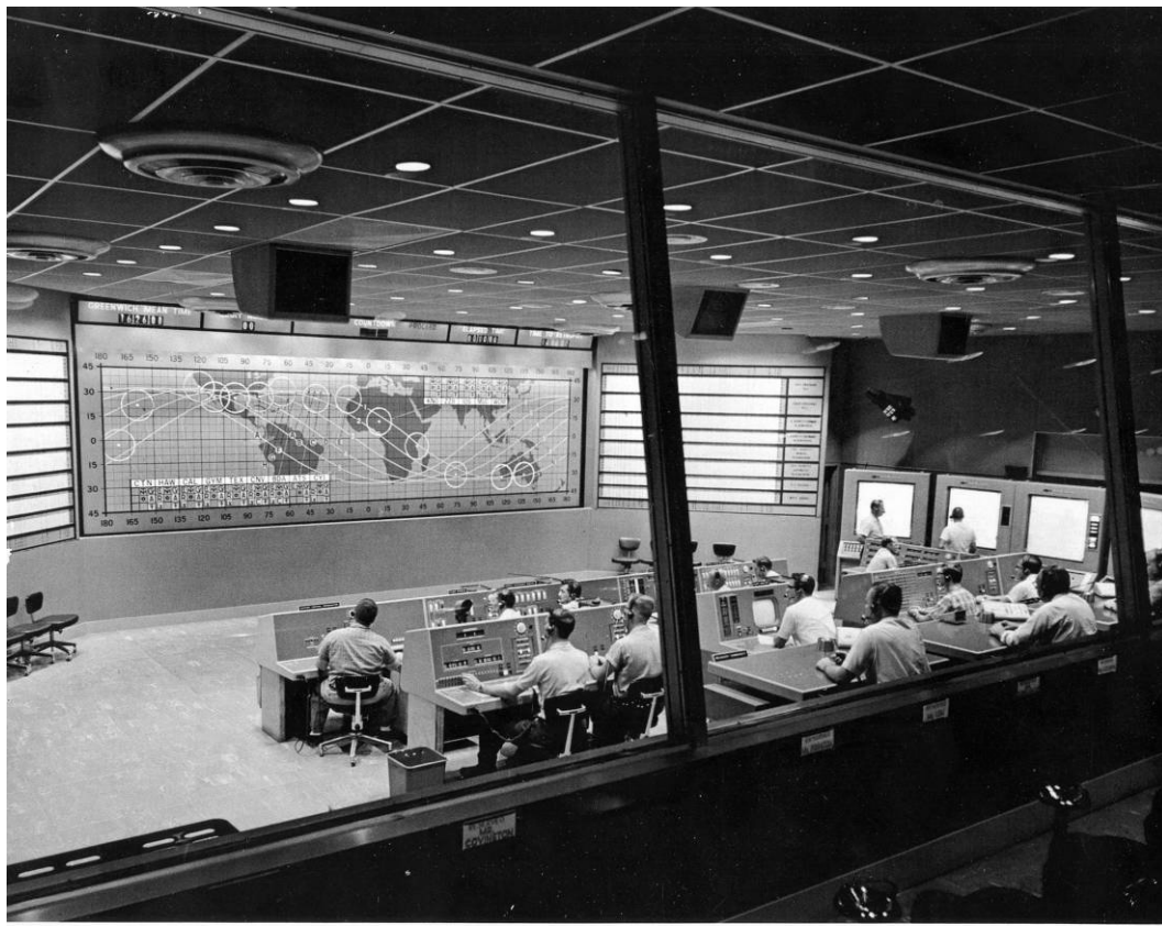
MA-8 MERCURY CONTROL CENTER
