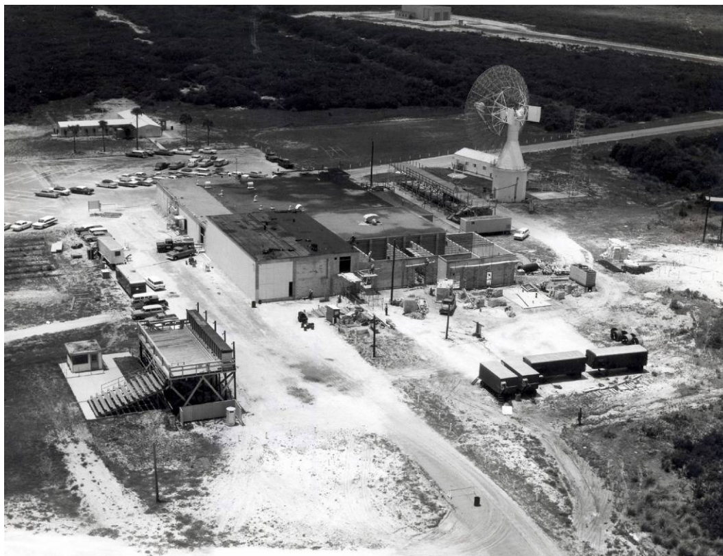
Figure A-2. Aerial view showing modifications to the MCC for Project Gemini, May 31, 1963. Source: John F. Kennedy Space Center, LOC-63-5634, on file KSC Archives.
