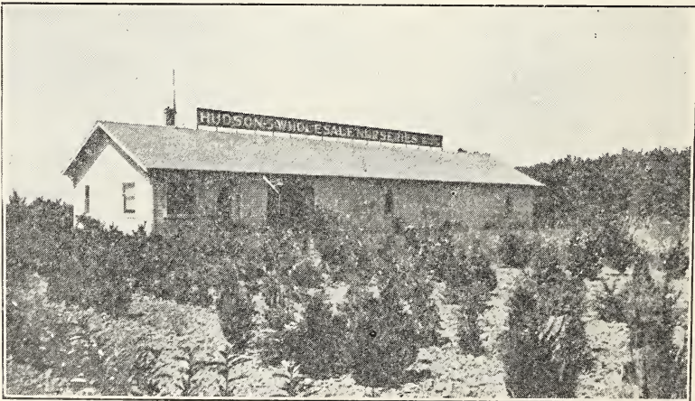
Office and Packing Building
