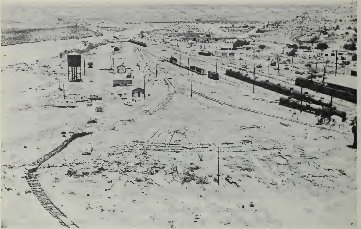
Aerial view, looking northwest, showing Southern Pacific railroad yard. Note damage to tracks and bridge approaches. Sanderson Canyon is in the left of the photo.
