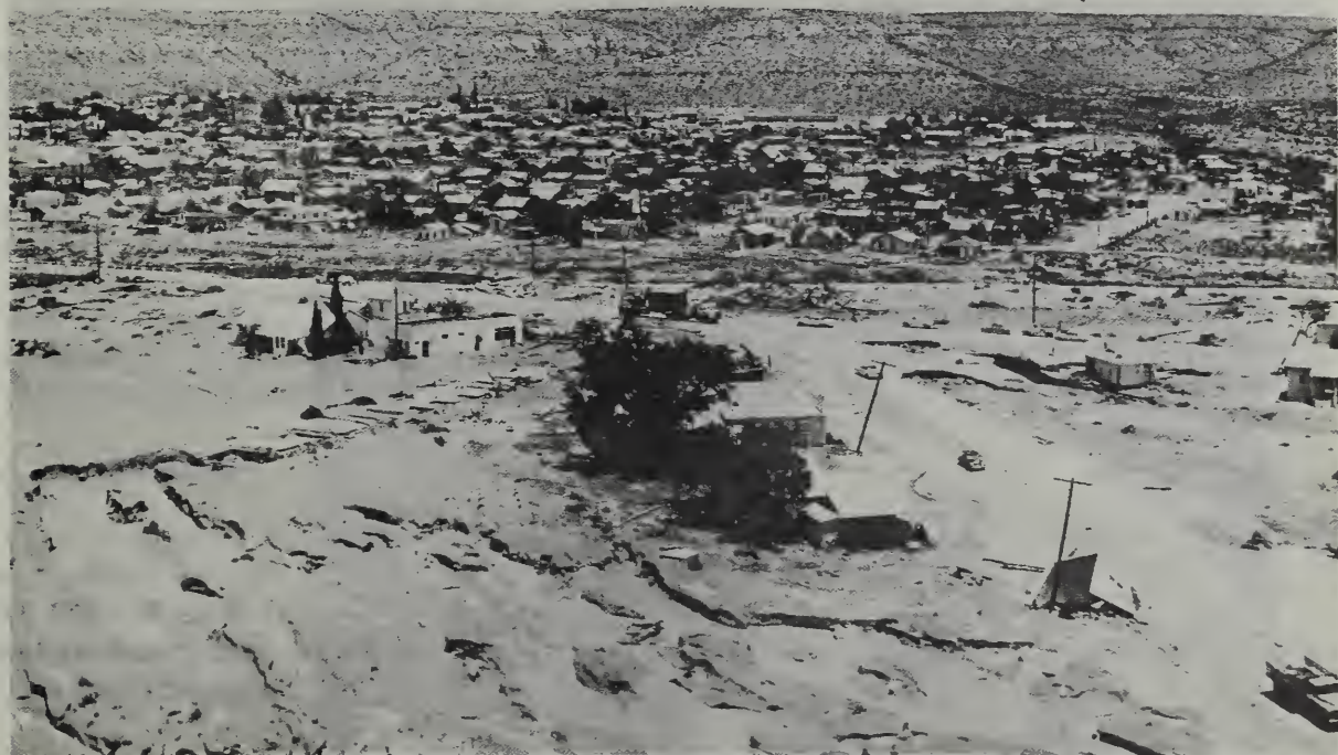
Aerial view of Sanderson. Note that foundations are all that remained of motel units destroyed by floodwaters. Several persons were swept away by the rushing waters.
