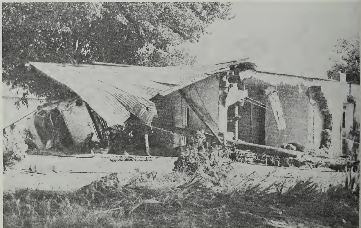
Raging waters destroyed this home. Adobe construction is typical of many of the homes in the urban area.
