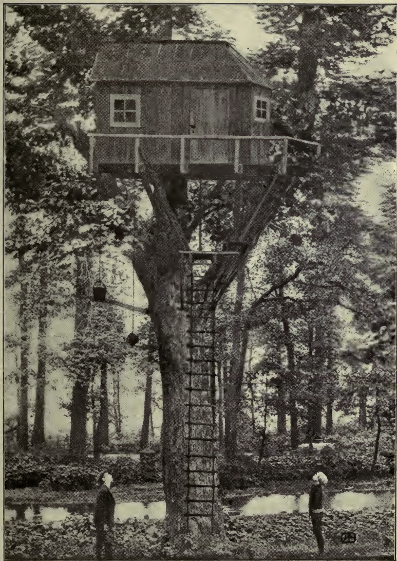
FIG. II—A SINGLE-TREE HUT
