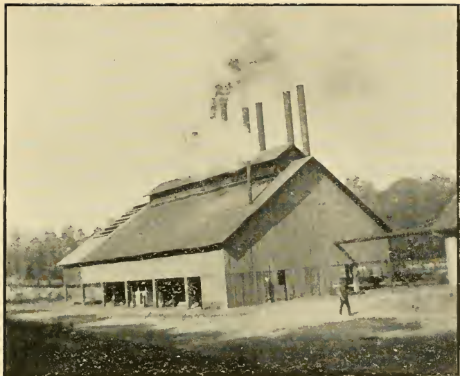
POWER HOUSE AT CONGO MINE.
