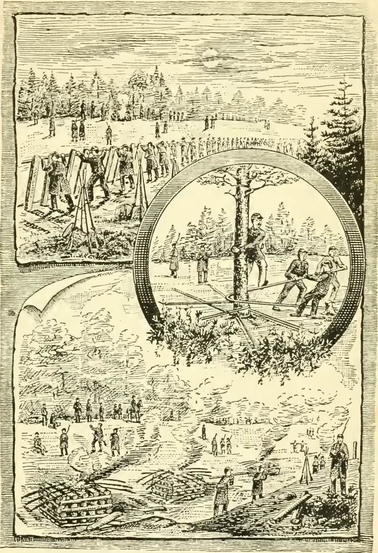
TEARING UP THE WELDON RAILROAD.
