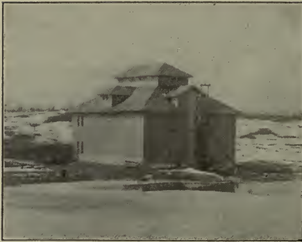
Fig. 79.—LOCAL COLD STORAGE
