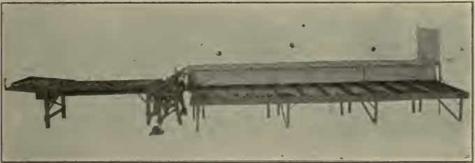
Fig. 24.—A GRADING MACHINE
