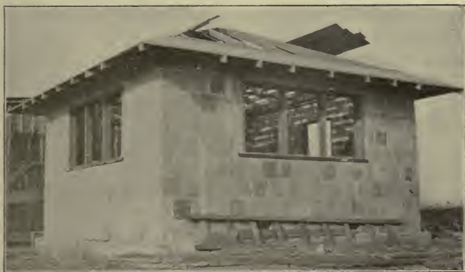
Fig. 78.—SMALL STORAGE AND PACKING-HOUSE
