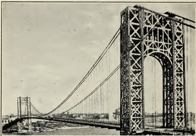
The strong cables of a great suspension bridge overcome the tremendous pull of gravity caused by the load on the bridge.
