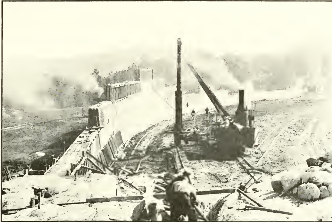
Close View of the Dam—1200 feet long, 85 feet high
