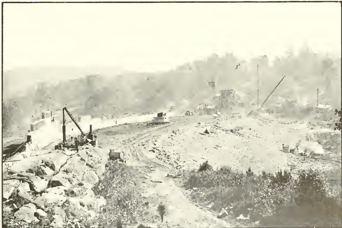
Birdseye View to show the immensity of the Job—Sept. 23, 1915
