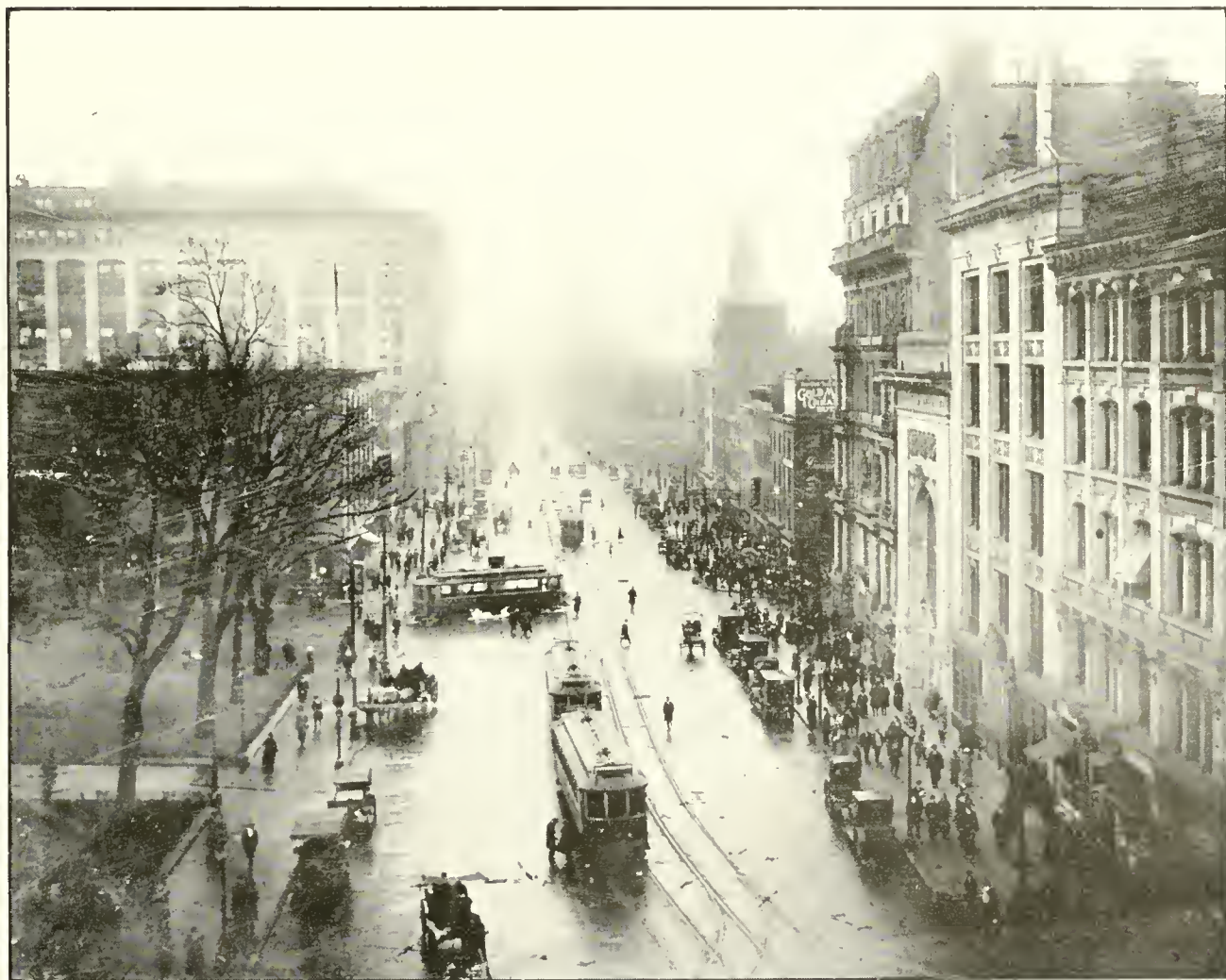
View of Main Street, Looking South
