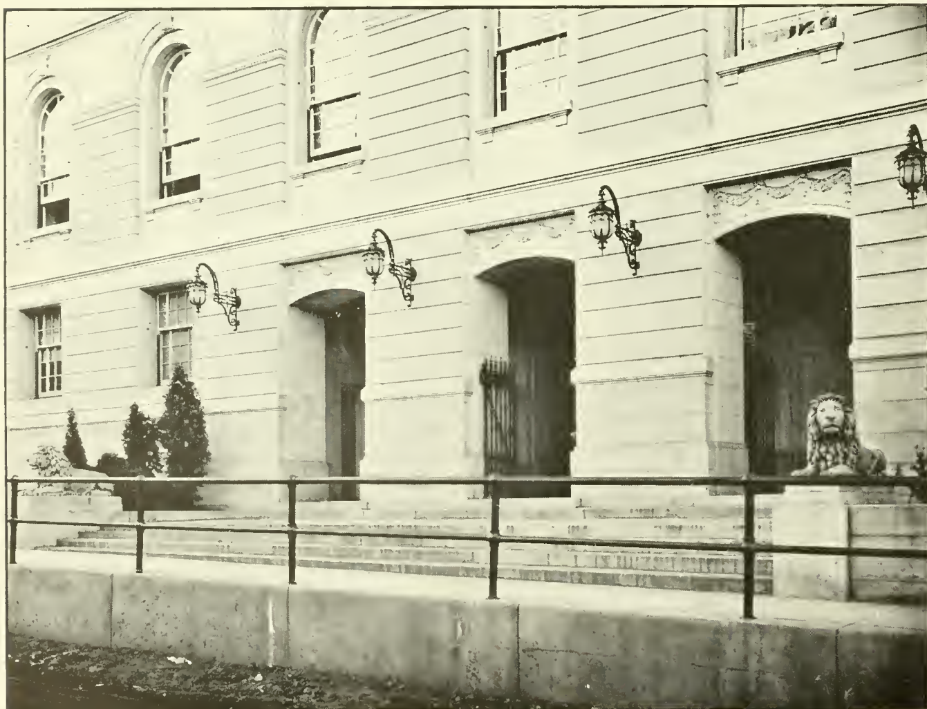
Arch Street Entrance
