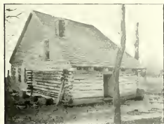
DOUGHTY'S CABIN, BUILT 1740.
