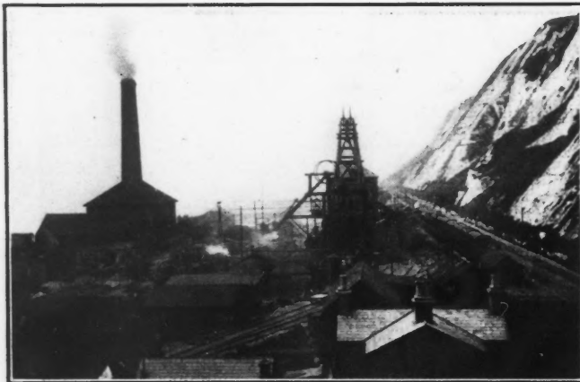
SURFACE WORKS, SHAKESPEARE CLIFF
