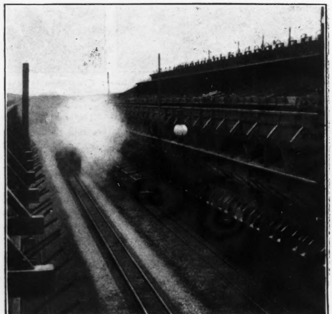
ORE CARS AT ORE-DRESSING BENCH
