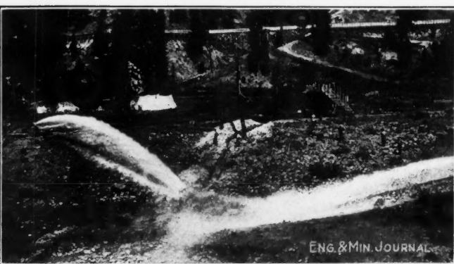
FIG. 6. GENERAL VIEW OF THE OPERATIONS
