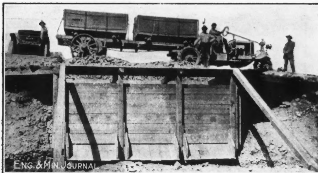
KNOX-MARTIN TRACTOR HAULING 15 TONS OF ORE IN SPECIAL DUMPING BODY
