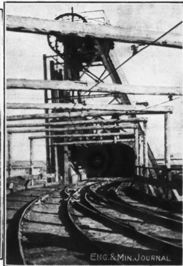
FIG. 9. HEADFRAME WITH BEGINNING OF TRESTLE
