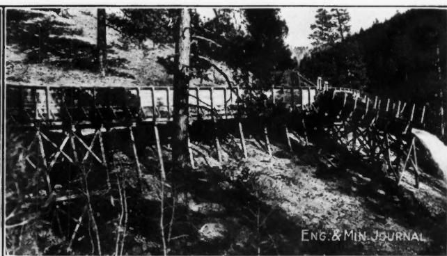
FIG. 4. A SPILLWAY IN THE FLUME
